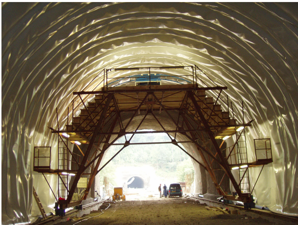
Tunel Krasíkov 2 - hydroizolace
