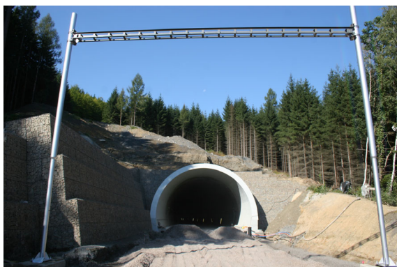
Tunel Malá Huba
